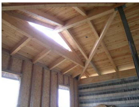
DETALLE VISTA INTERIOR
